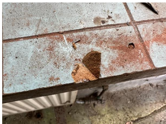
Vensterbank is van hout
